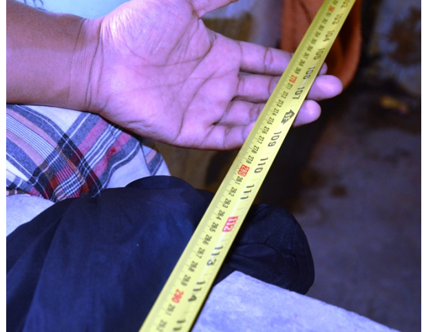
Taking measurements of the existing floor tank which will be modified to serve as a rainwater collecting tank
