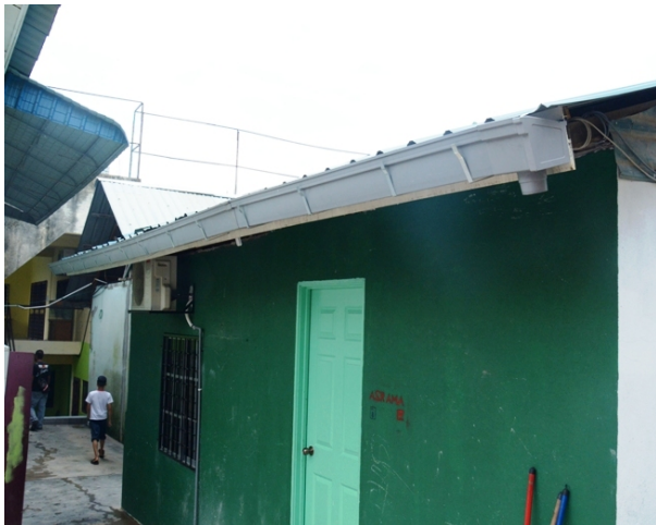
The gutter installed at a building near the washroom
