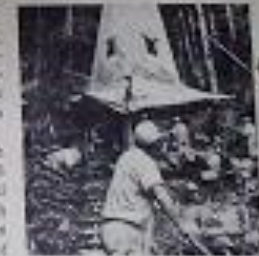
Exploration drilling to obtain rock sample for examination
